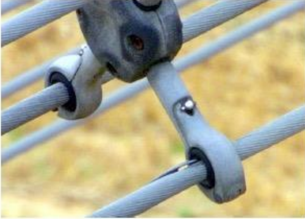
Overhead line showing signs of deterioration.
