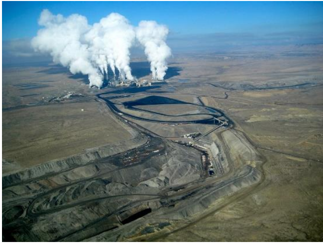
View of San Juan generating station and mine coal piles
