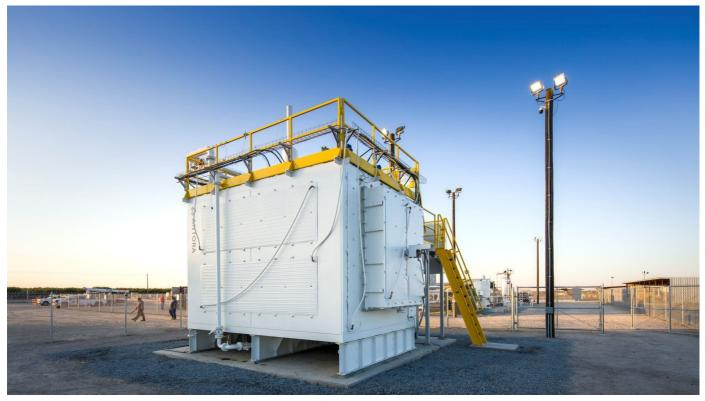
The Antora thermal energy storage battery uses graphite as a heat storage material with temperatures reaching 1,800°C
